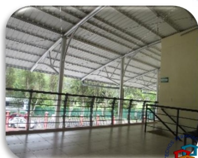
TERMINAL BUS JINOTEGA
